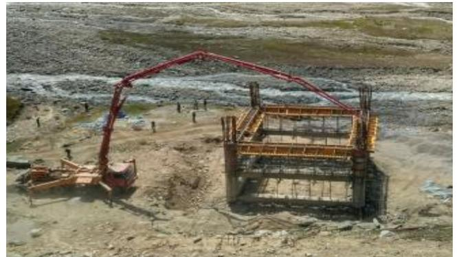
Fig 23. Casting of foundation
