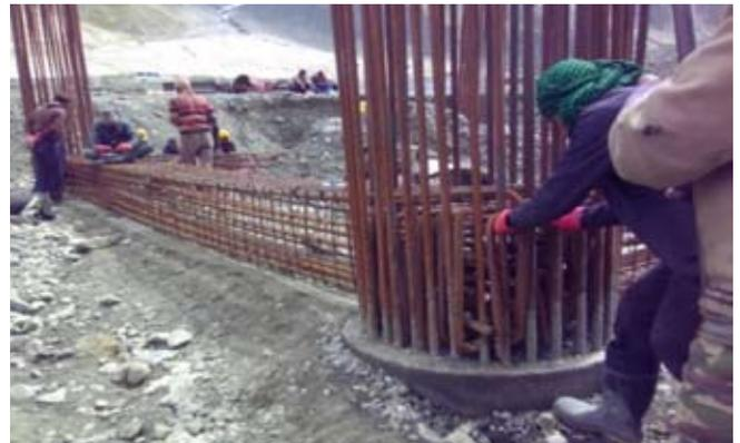
Fig 21. Reinforcement bar tying
