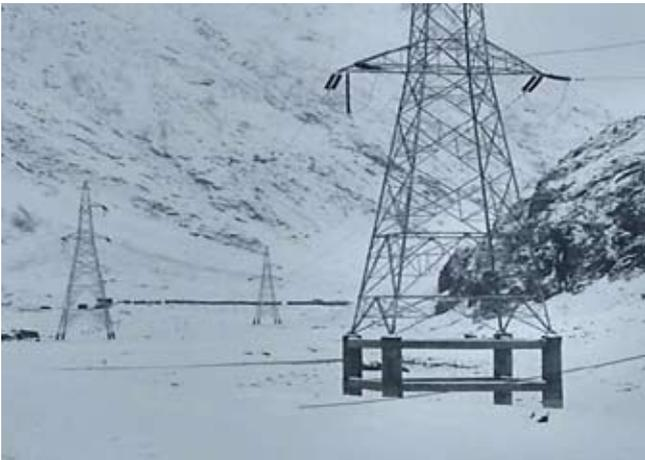
**Fig 5.** Raised Chimneys for increased clearance for conductors
